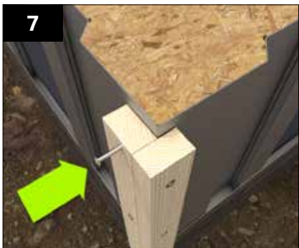
At corners battens should be fixed as shown. This ensures that claddings at the corners are well reinforced.
