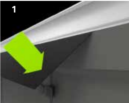
If glass roof fold the EPDM over the walling membrane.
