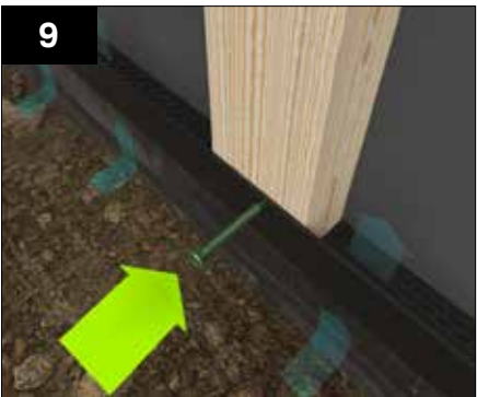
At the base of the wall attach the perforated ventilation trim to the battens. This allows for ventilation and drainage but inhibit vermin/insects. (Except for Brick Slip Rail (go to page 37), where the starter rail replaces this part)
