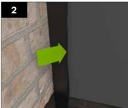
At the host wall fold the vertical DPC over the top of the membrane prior to battening out.
